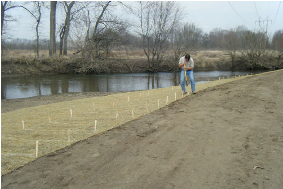
3/16/2009 12:40:20 PM# Leighann Gerardi McCulla at Honeycreek restoration_5.JPG
