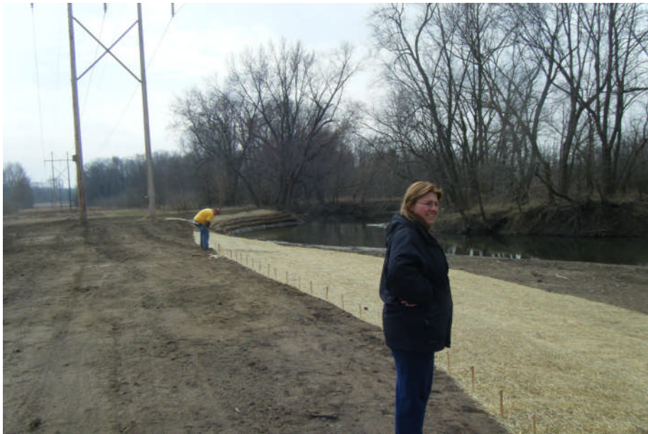
3/16/2009 12:36:05 PM# Leighann Gerardi McCulla at Honeycreek restoration_1.JPG
