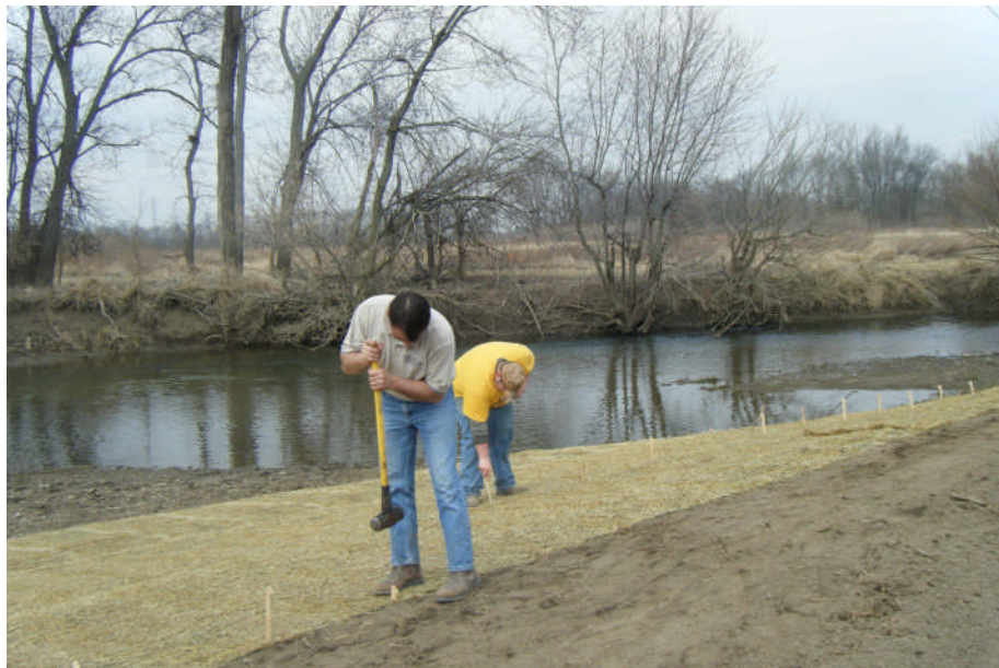
3/16/2009 12:38:42 PM# Leighann Gerardi McCulla at Honeycreek restoration_4.JPG
